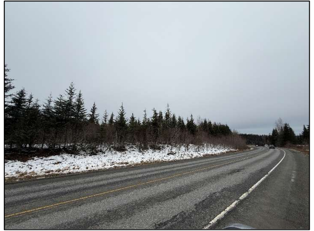
Looking west from Sterling Highway viewing excess land
