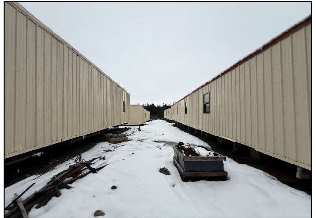
Looking at the south and north sides of Building Administration/Barrack Buildings
