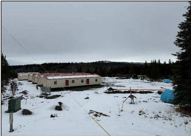
Looking at the south and west side of buildings from Old Sterling Highway
