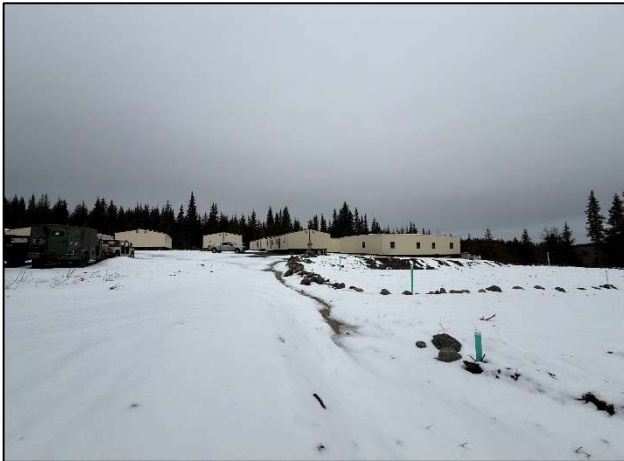
Looking at Septic Leach Field
