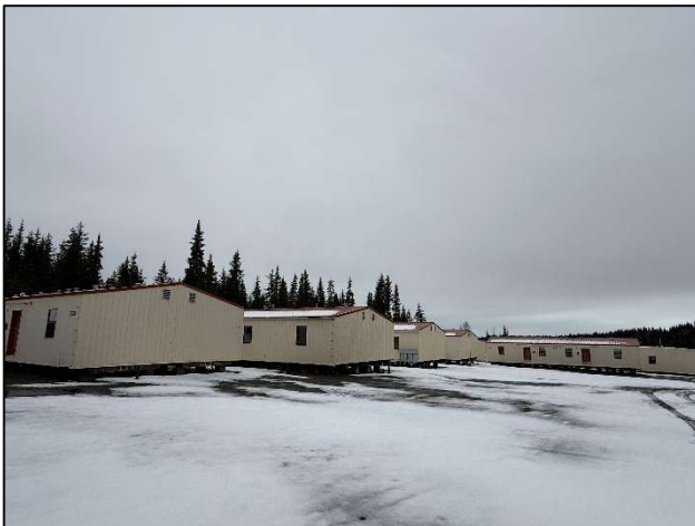
Looking at the south and east side of buildings from Old Sterling Highway
