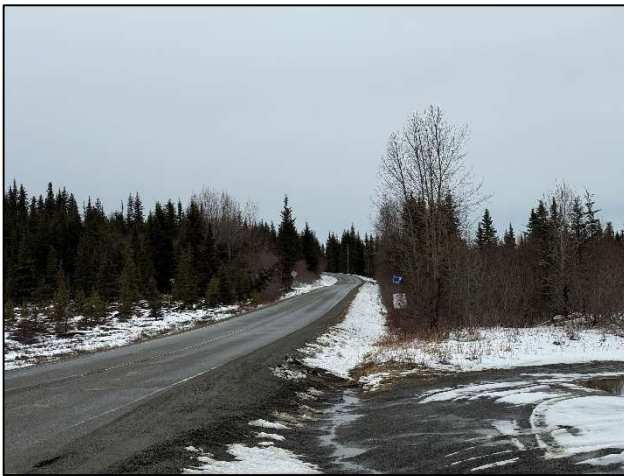
Facing northwest along Sterling Highway Subject at right
