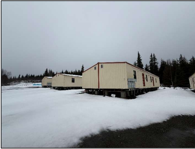
Looking at north and east of buildings Barrack Buildings
