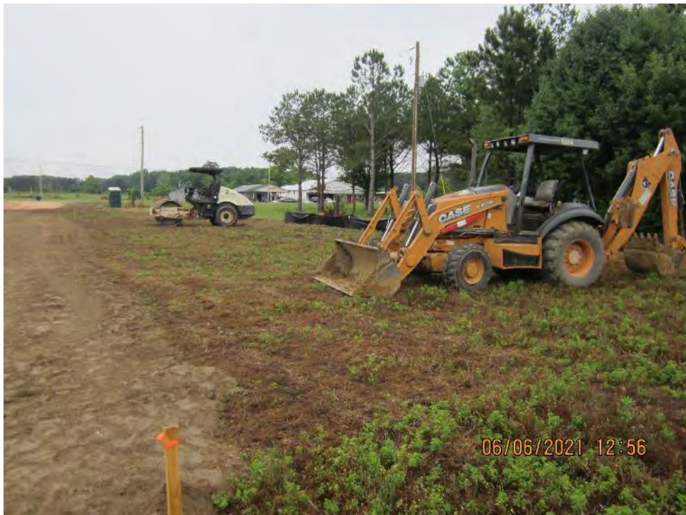
Photograph 8: View of construction equipment temporarily located on the east portion of the subject site for site-grading operations currently in progress.
