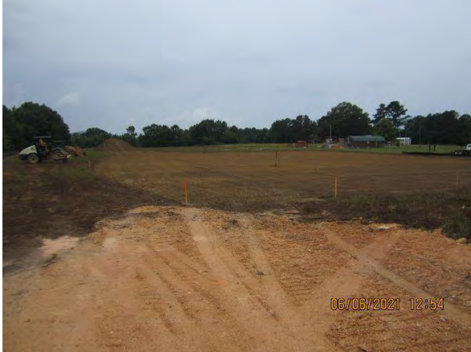
Photograph 3: South view of the northeast portion of the subject site.
