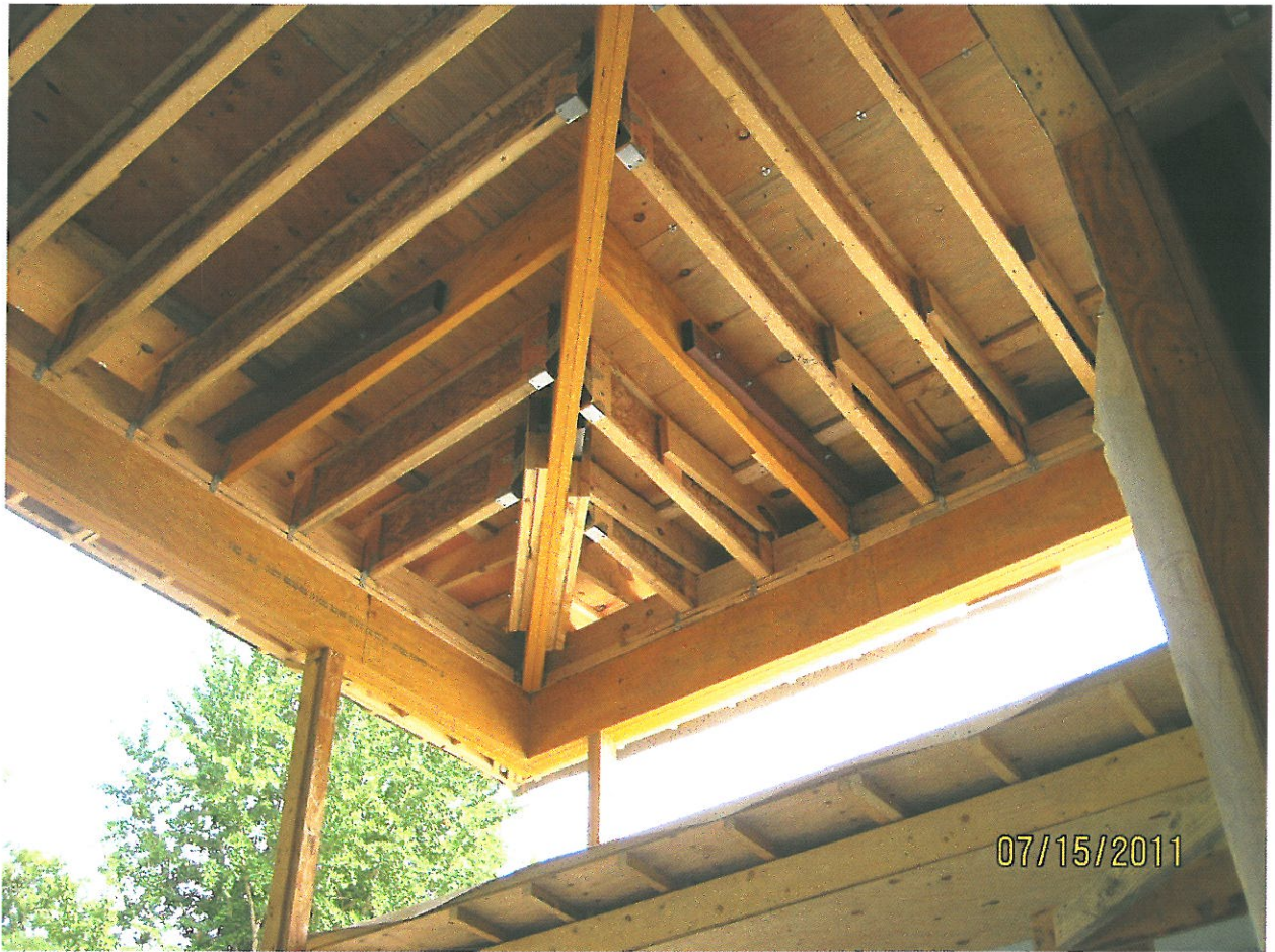
Photograph 9: Roof tube framing.
