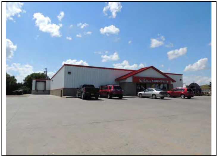
8. Looking west – Linton Food Center is located north of Scherr’s Meats (a north adjoining property).
