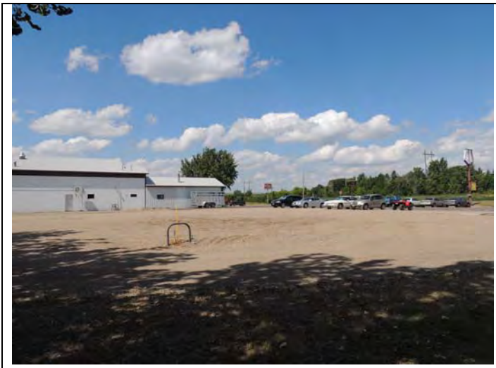
3. Looking north – View of the Site property.
