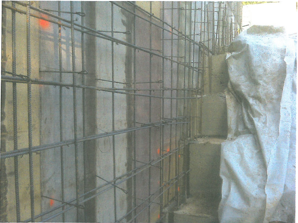
Photograph 1: Reinforcing for the concrete basement walls.
