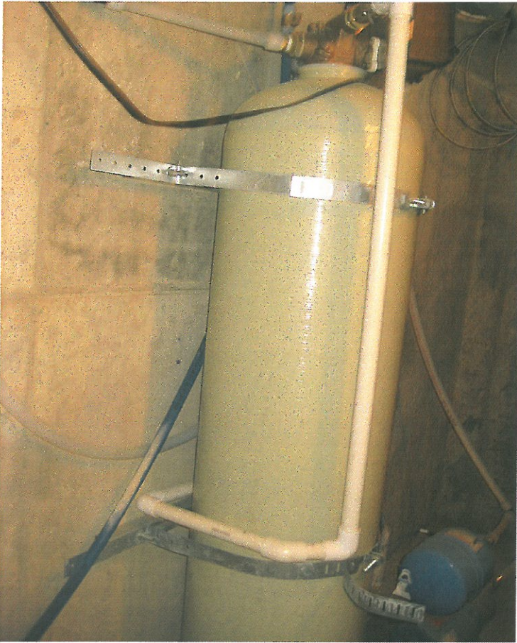
Photograph 7: Tank strapping.
