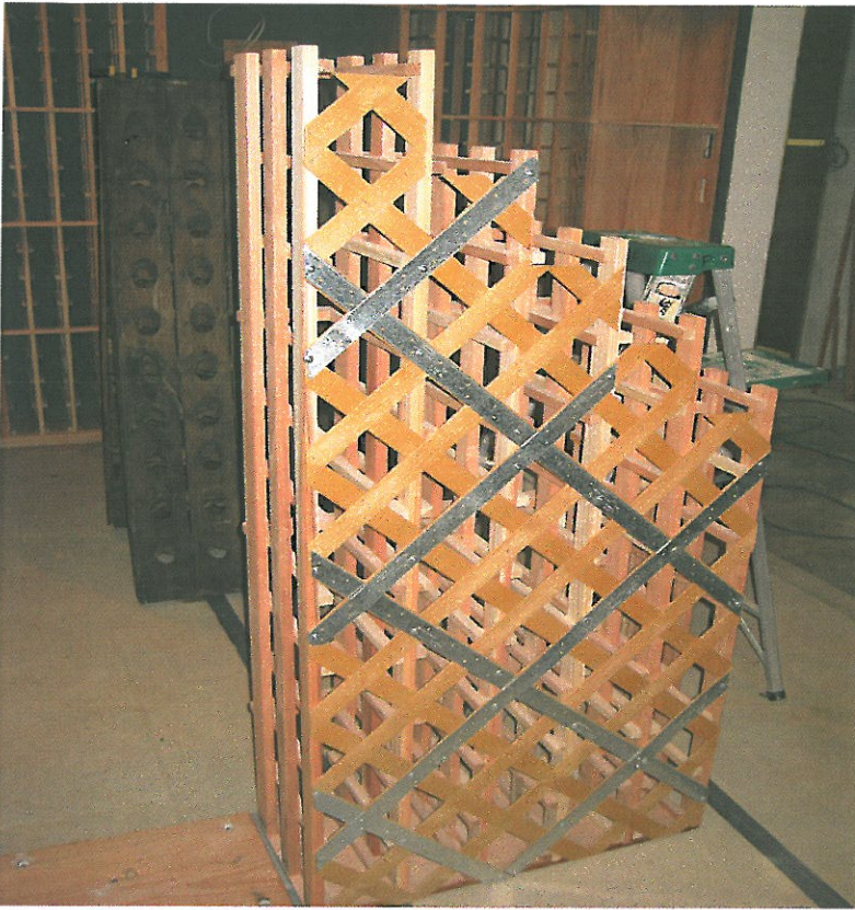
Photograph 3: Wine rack strapping.
