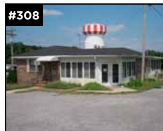
#308 18260 Hwy 31 N, Vinemont Commercial building that was once occupied by a beauty shop.
